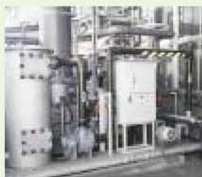
Remediation procedure at the Main Factory
