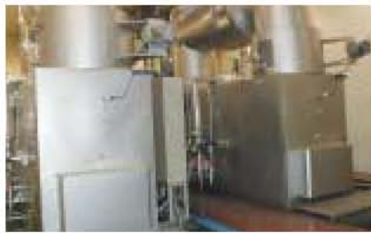
Newly installed cogeneration system (Yamaha Metanix Corporation)
