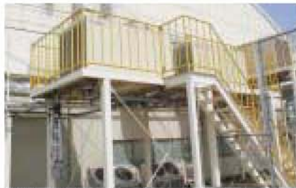
Outside air latent heat processing system that produces higher-efficiency air-conditioning (Tenryu Factory)
