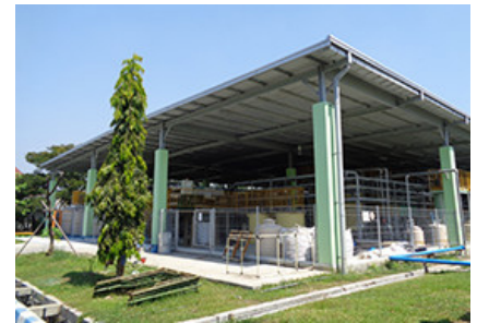
Wastewater treatment facility at YMPI
