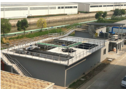
Wastewater treatment facility (Hangzhou Yamaha)
