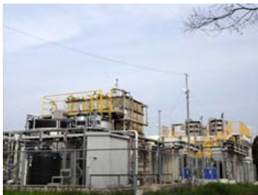
Wastewater treatment facility at the Kakegawa Factory
