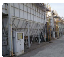
▲ Dust collection equipment (Hangzhou Yamaha Musical Instruments Co., Ltd.)
