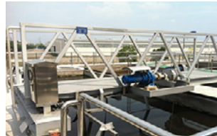
Reuse of wastewater for cooling water (Hangzhou Yamaha Musical Instruments)
