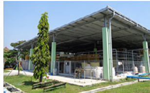
Wastewater treatment facility (Yamaha Musical Products Indonesia)
