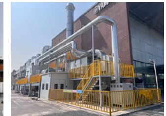
VOC treatment facility (Xiaoshan Yamaha Musical Instruments)
