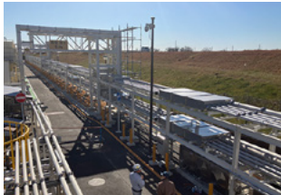
Redoubling of leak and general inspections entailing unearthing of wastewater pipes installed in underground tunnels
