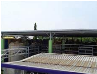
Wastewater treatment facility at YMPI
