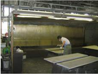
Wet painting booth(Kakegawa Factory)
