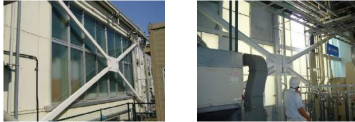
Improving earthquake resistance at the Toyooka Factory
