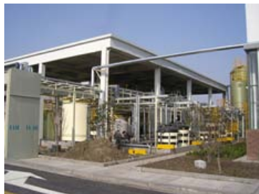
Wastewater treatment facility
