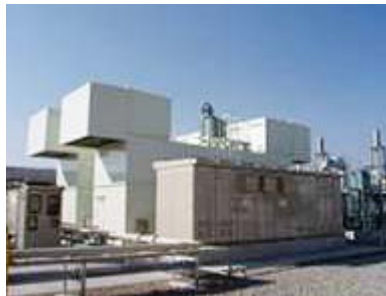
Cogeneration system facility
