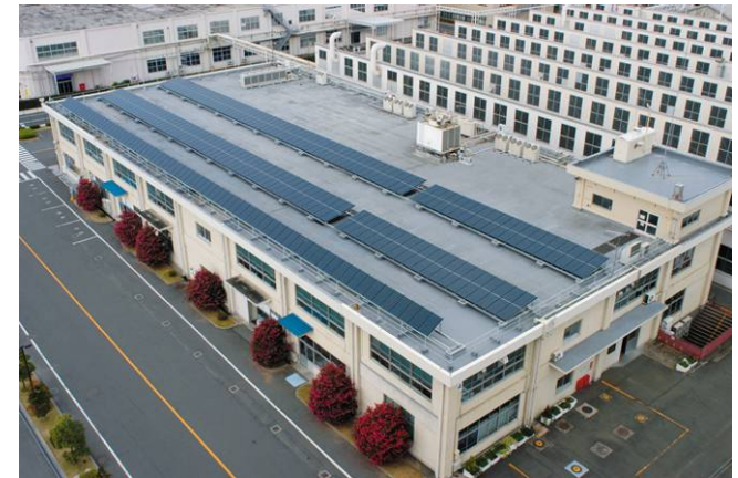
solar power generation device
