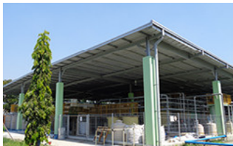
Wastewater treatment facility
