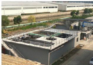
Wastewater treatment facility
