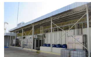
Wastewater treatment facility
