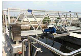
Reuse of wastewater for cooling water
