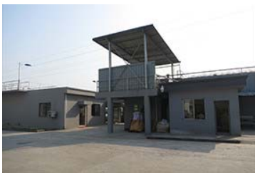
Wastewater treatment facility (Hangzhou Yamaha)
