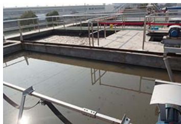
Reusing wastewater for cooling water (Hangzhou Yamaha)
