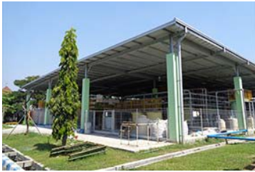
Wastewater treatment facility at YMPI
