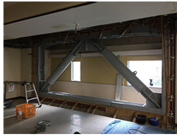
Improving earthquake resistance at a Nagoya business site
