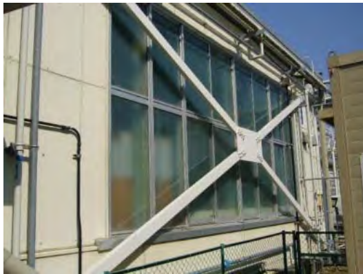
Improving earthquake resistance at the Toyooka Factory
