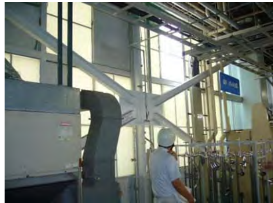
Improving earthquake resistance at the Toyooka Factory
