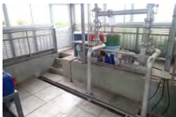
Circulating water tank for painting booths (Xiaoshan Yamaha Musical Instrument Co., Ltd.)
