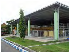
Wastewater treatment facility at YMPI
