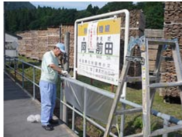
Painting guardrails at the Ani-Maeda Station
