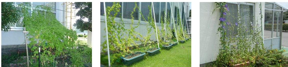
Green Eco Curtain at Yamaha Corporation's headquarters office
