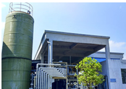
Wastewater treatment facility
