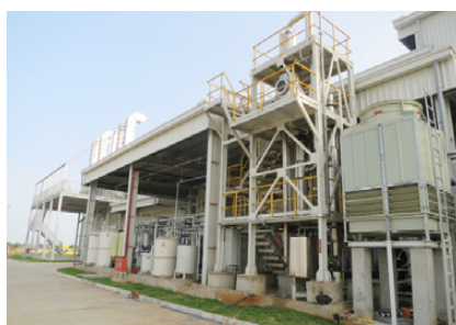
Wastewater treatment facility
