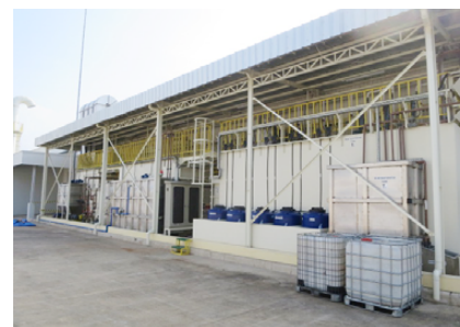
Wastewater treatment facility
