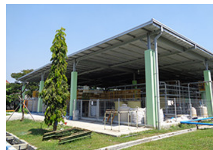
Wastewater treatment facility
