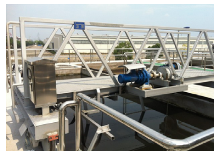
Reuse of wastewater for cooling water
