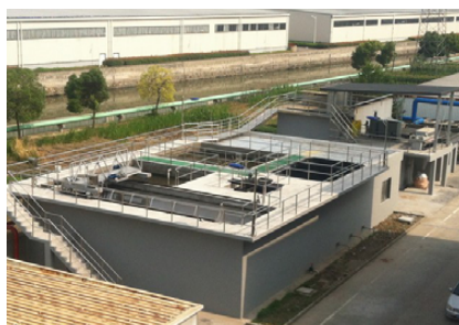
Wastewater treatment facility
