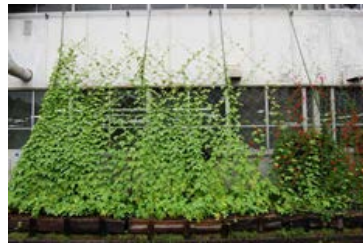
Green Eco Curtain at the Saitama Factory
